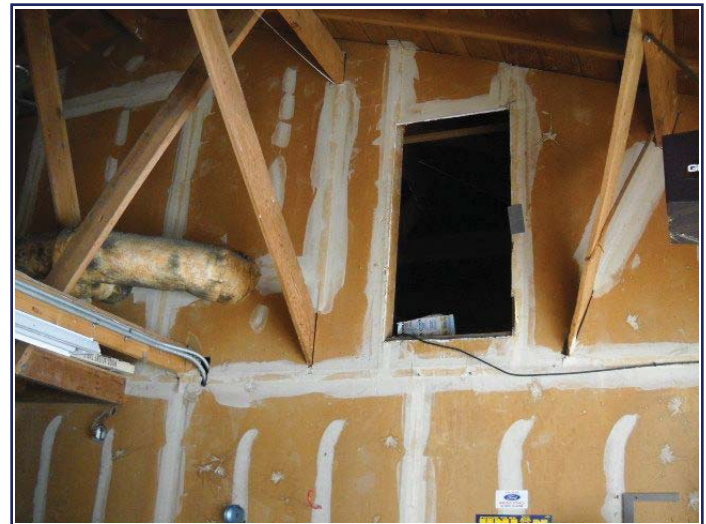
Open access to the attic.
